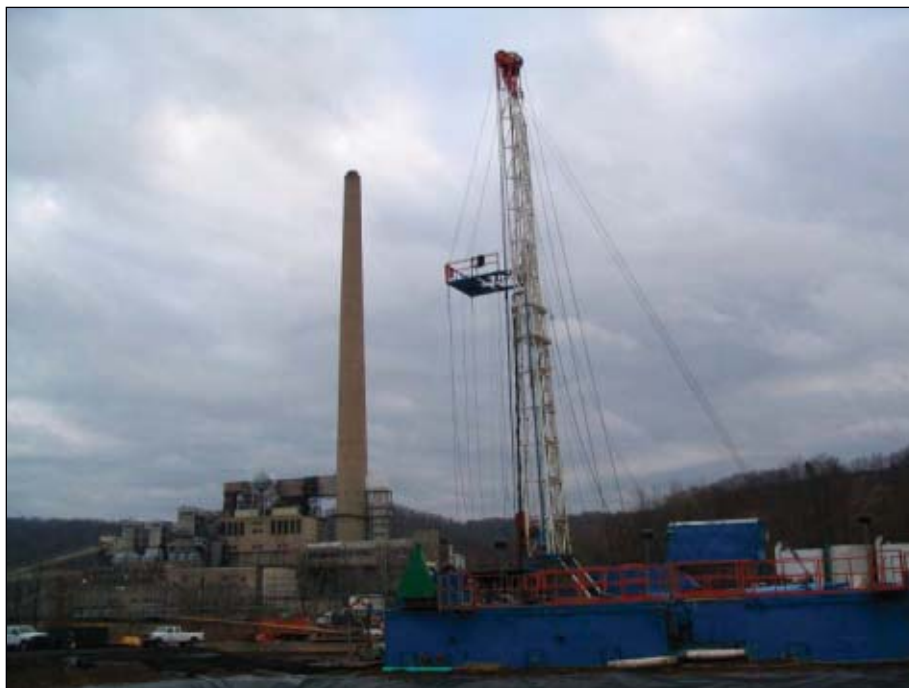
Through the Midwest Regional Carbon Sequestration Partnership, Battelle scientists drilled an 8,000 ft test well at First Energy's R.E. Burger Plant near Shadyside, Ohio, to evaluate CO 2 storage potential in Appalachian basin. Drilling was completed in February. Photo from Battelle.
